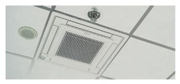
The FFA-A2VEB's new panels have been designed to integrate with standard ceiling tile dimensions, enabling lights, so it's easy to install a Daikin Fully Flat Cassette, and speakers and sprinklers to be in stalled in the adjoining ceiling tiles.
